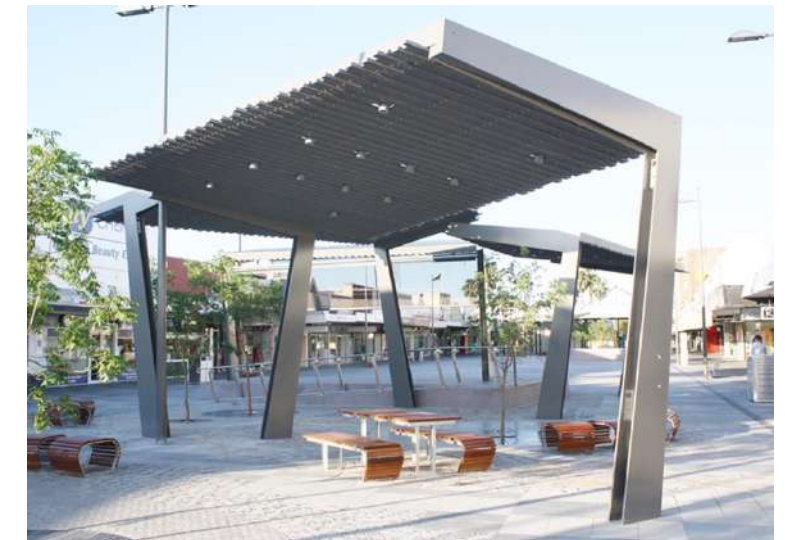
Shade structures with recycled plastic. Source: Integrated Recycling
