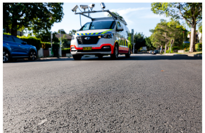
Paving the Way: The Reusing Rubber - Recycling Tyres for Roads works phase is complete.
